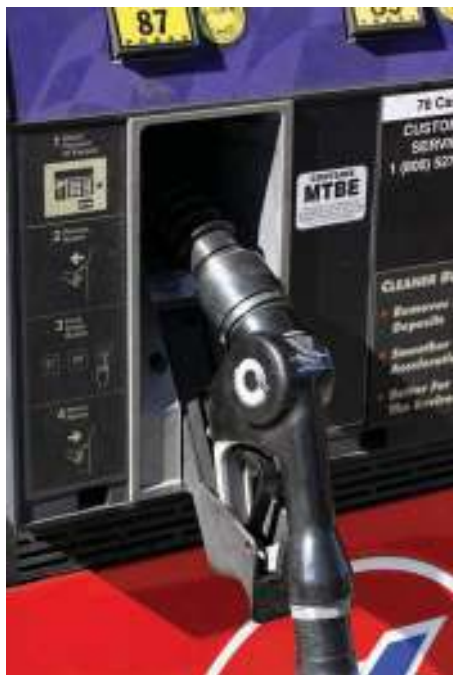
▲ MTBE is a component of some gasolines but is being phased out because it has been found to be an unsafe contaminant of groundwater.
