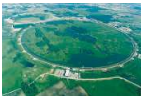
▲ The Fermi National Accelerator Laboratory has a particle accelerator 4 mi in circumference that is able to accelerate protons to energies of 1 trillion eV.
