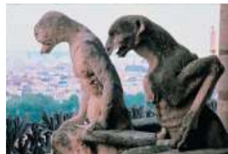
▲ The details on this marble statue have been eaten away over the years by acid rain.
